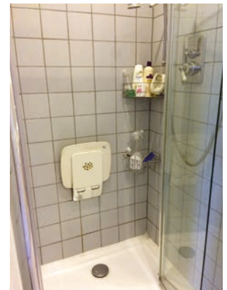
A level access shower can be easier to use than a bath. Note the flip-down seat on the wall.
