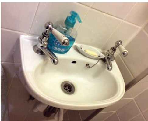
Lever taps on all sinks and basins are much easier to use than knobs
