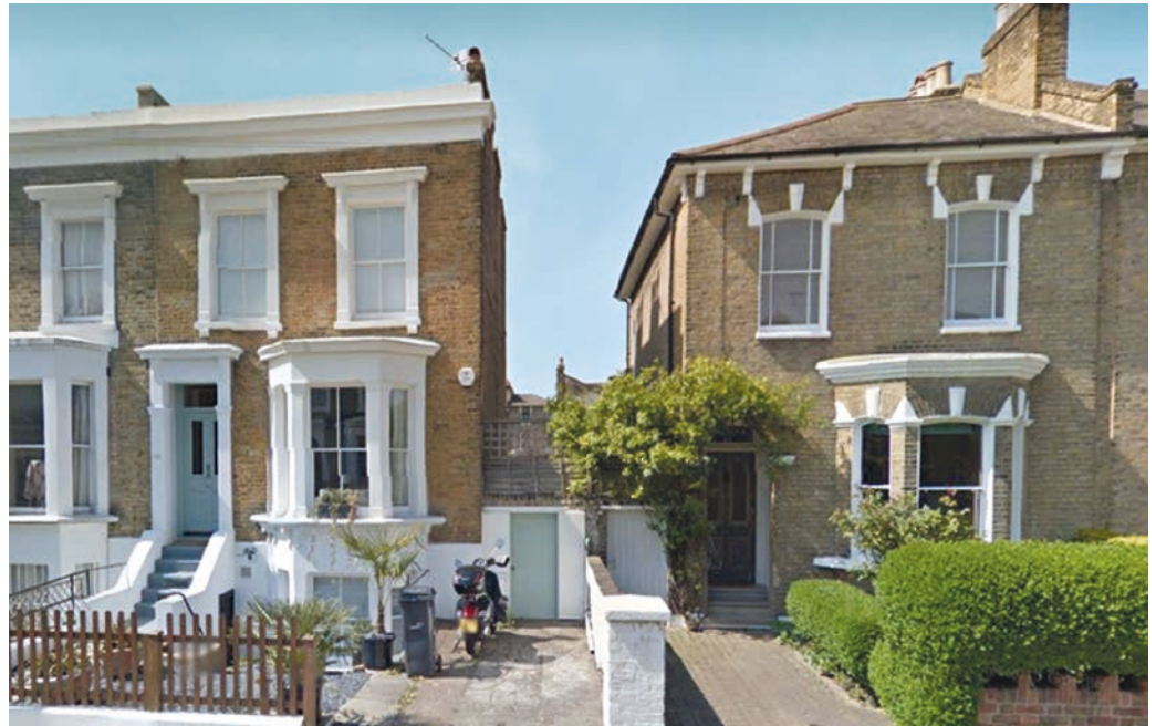
Two Victorian houses: on the left, steps up to the raised ground floor and down to the basement. On the right, three steps into the house
