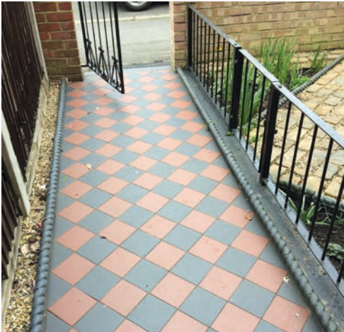
A new ramp rises from the pavement up to the front door to eliminate steps
